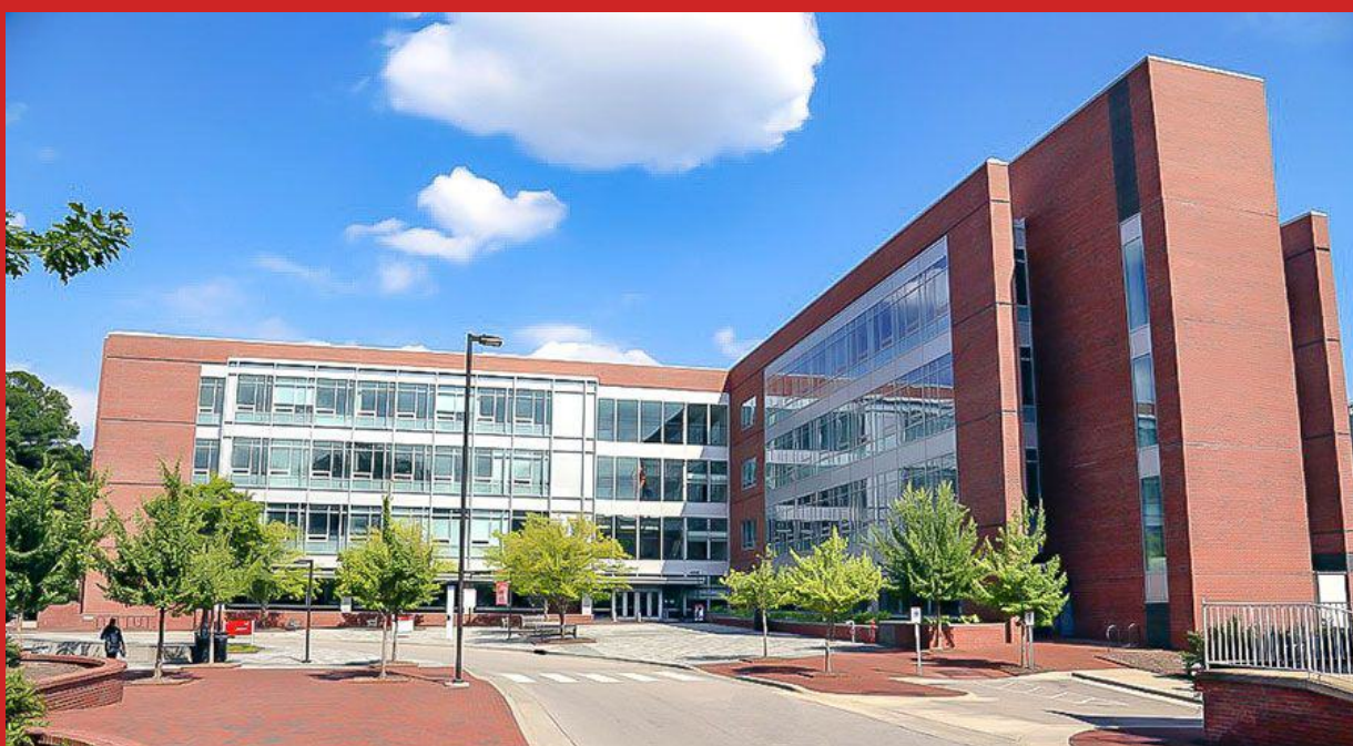
SAS Hall at NCSU's Main Campus
